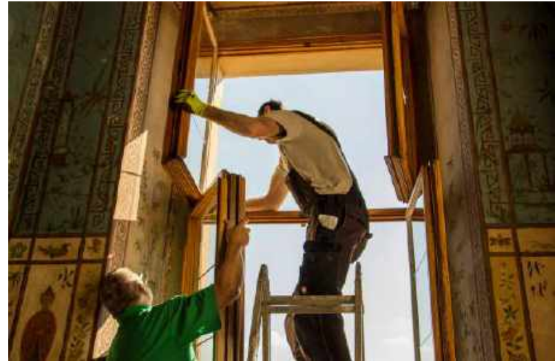
Installation of new replicas of original Renaissance windows.
