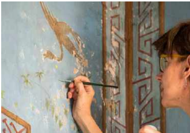
(left to right) Restorer Ilona Chlubnová cleaning dust and dirt, ironing on loose layers, retouching wall paintings, and filling in cracks in the wall by injecting them with plaster.
