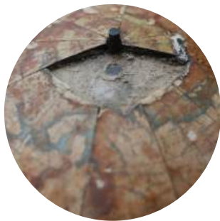
Detail of a severe damage.
